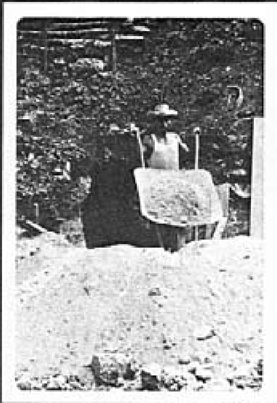
Photo 6 Guatemalan workman excavating tunnel between Strs. 50-72 and -73.
