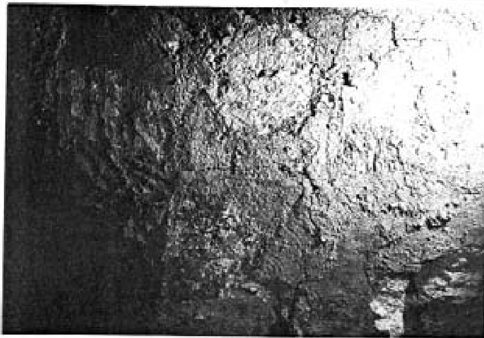
Photo 26 Su. 196, drip lines of vault mortar.
