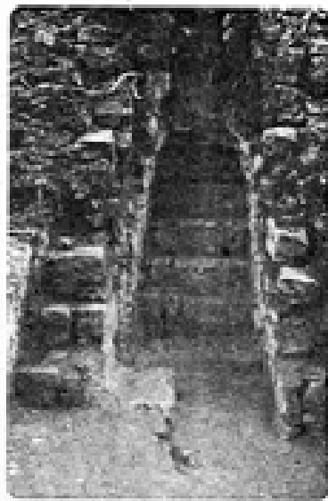
b) 1st masons' stair
