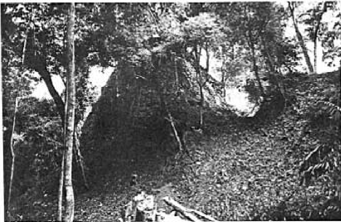
Photo 5 Rear of Str.5D-73 after bushing but before excavation.
