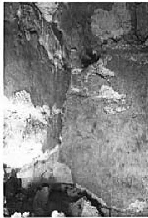
Photo 21 Sta. 106, southeast corner showing joints of vault mortar caught by cloth draped over east wall from east look.
