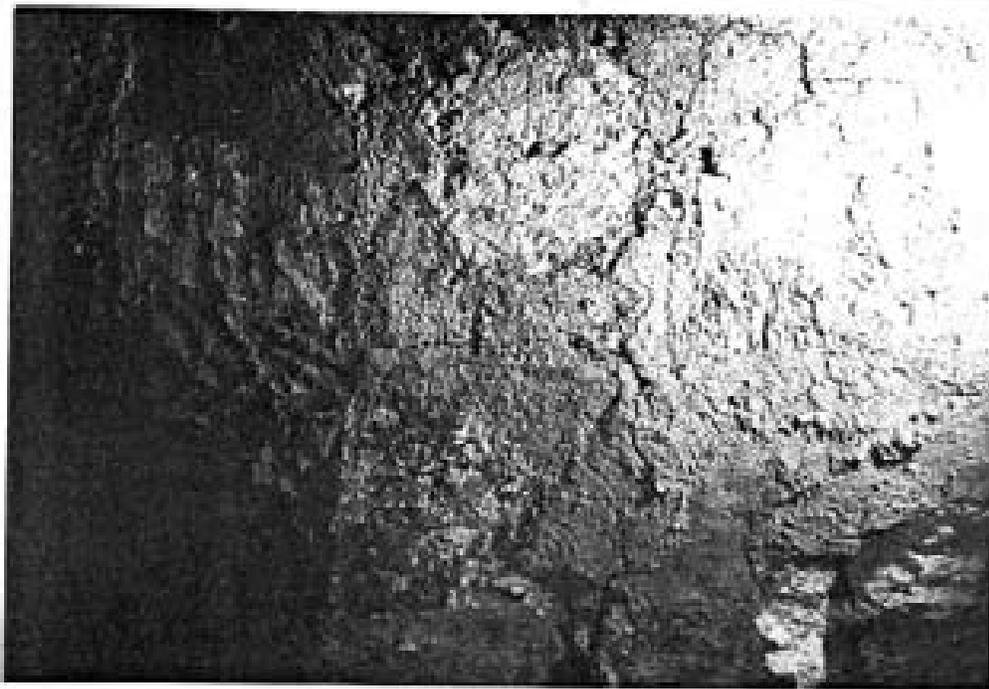
Photo 26 Su. 196, drip lines of vault mortar.
